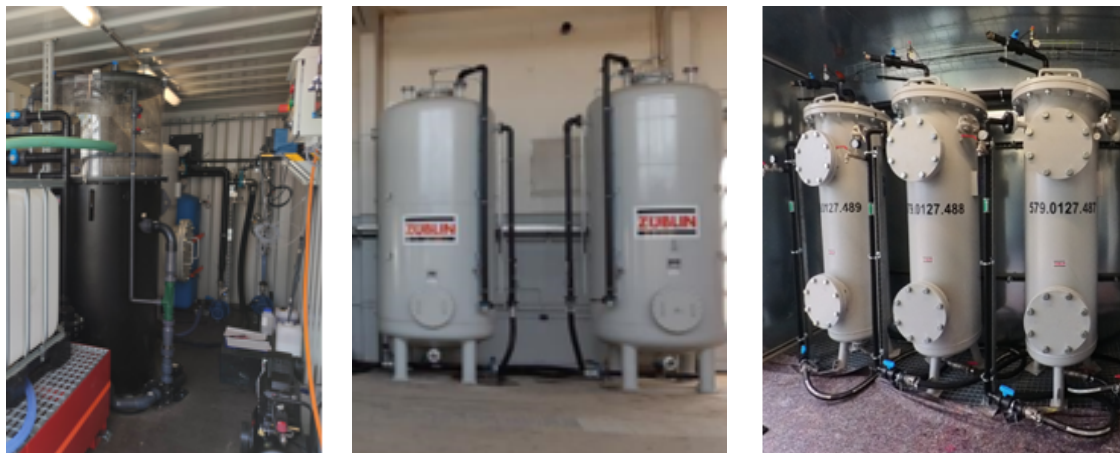
Fig. 3: Apparatus for efficient PFAS removal: Foam fractionation (left), Activated carbon adsorption (centre), Ion exchange (right)
