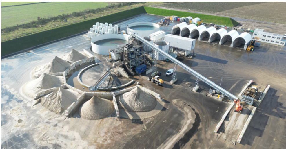
Fig. 1: Soil washing plant for PFAS-contaminated soils in Northern Germany, throughput approx. 2,000 tonnes of soil/d, integrated process/sludge water treatment
