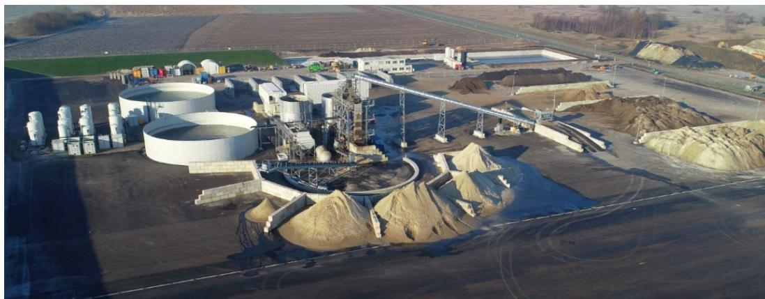
**Fig. 2:** Soil washing plant for PFAS contaminated soil in Northern Germany.
