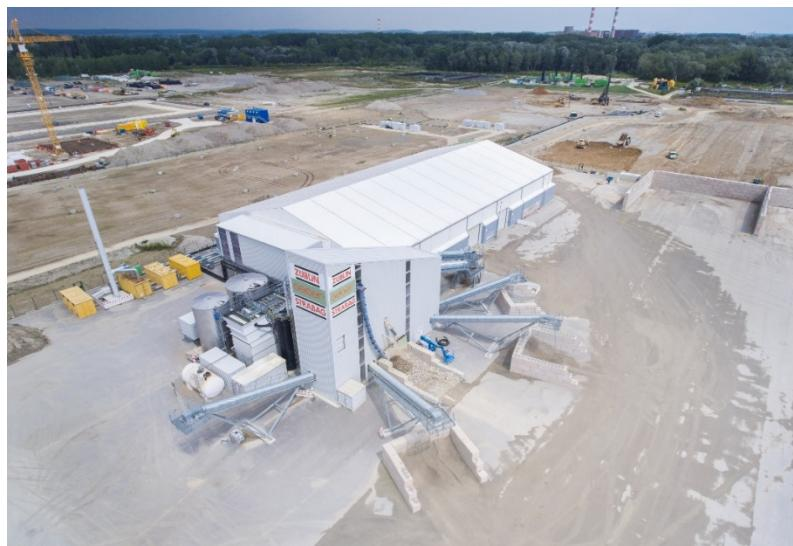
**Fig. 1:** Soil washing plant for PFAS and HC contaminated soil at the site of a former oil refinery in Southern Germany
