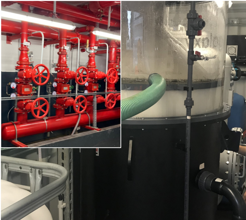
Sprinkler system - foam fractionation unit
