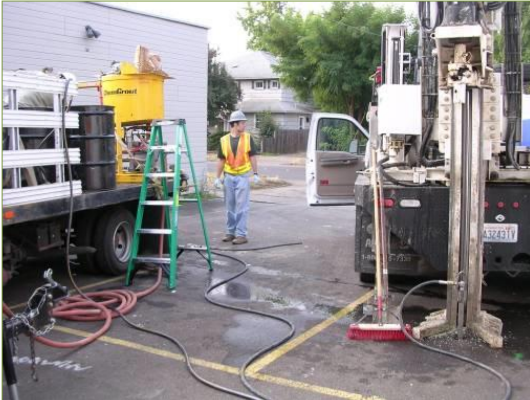
ChemGrout's CG-550 mixing and injection unit
