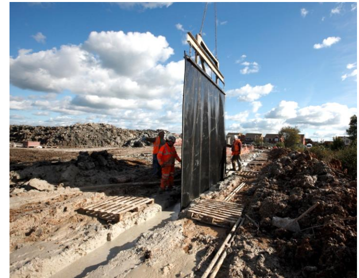
Cut-off wall with membrane, landfill containment, United Kingdom
