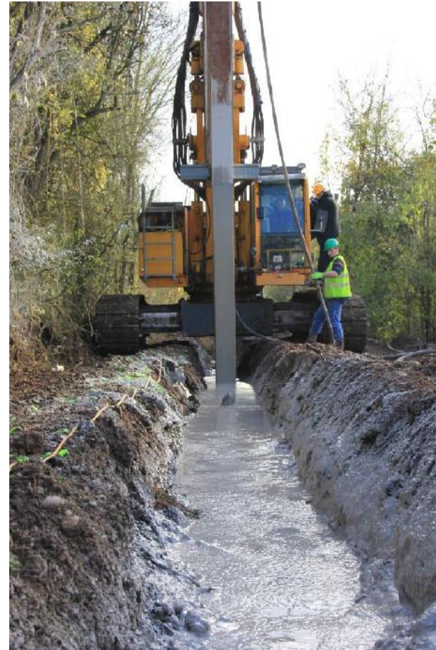
Cut-off wall with vibrated profile, dike in France
