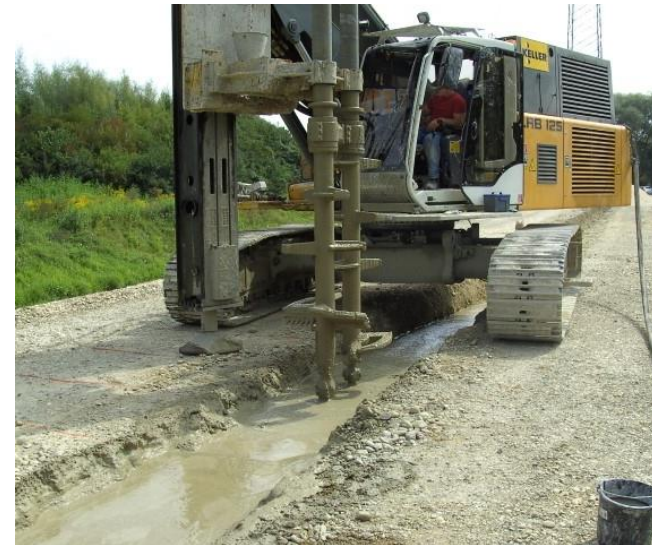
Cut-off wall with DSM, dike in Germany
