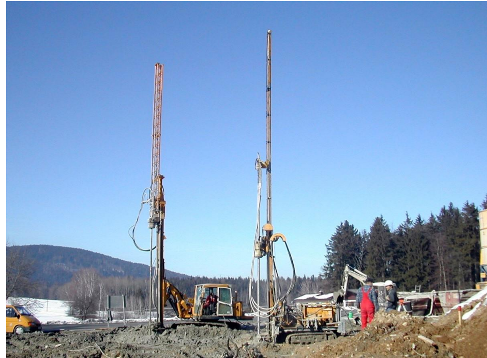
Immobilization of oil pollution with jet grouting, gas station in Austria
