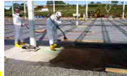
Figure 4-1. Liquid Boot® being applied during construction. Courtesy LBI Technologies, Inc.
