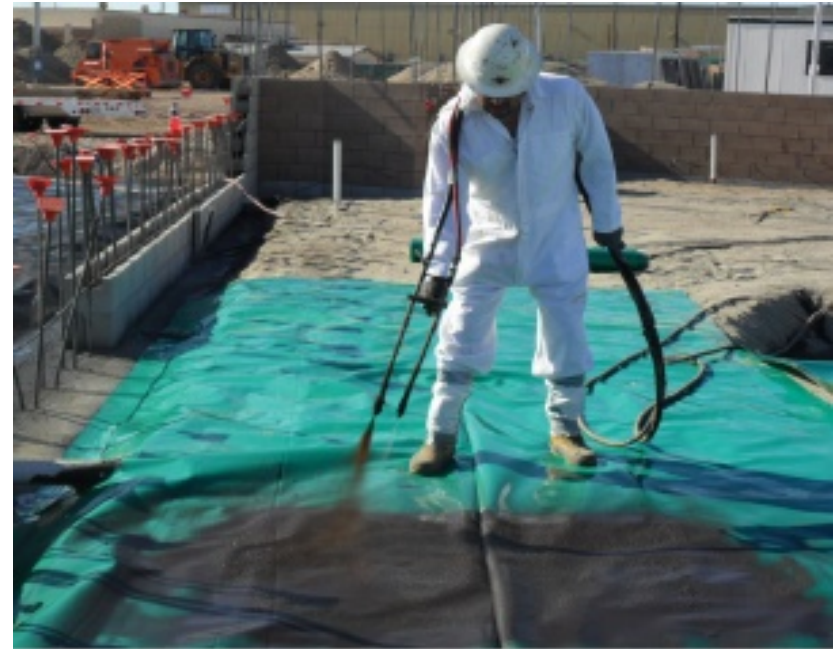
Liquid Boot™ polychloroprene latex-asphalt emulsion being spray applied
