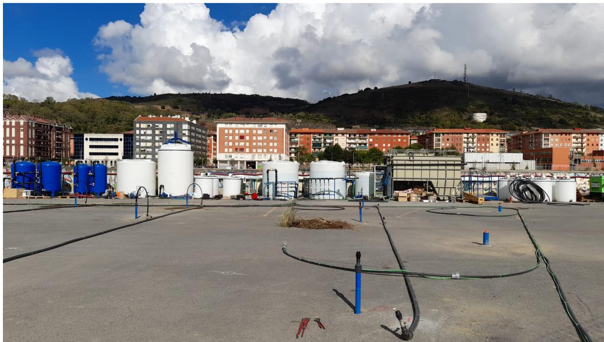
The plant is designed to perform (i) soil conditioning and hydro-chemical-microfracturing, to improve permeability and facilitate the diffusion of treatment fluids, (ii) biostimulation, (iii) bioaugmentation with selected biomass (fungi and bacteria), (iv) chemical flushing of inorganic contaminants and (v) extraction and purification by physio-chemical treatment and filtration of contaminated groundwater.
